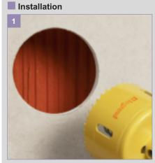
Hole cutter saw Ø67 Box Ø67 mm, more space for cabling
